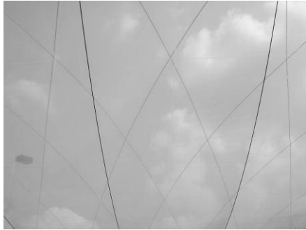
3.1 Large-format ETFE-cushion to look through, source Cenotec
