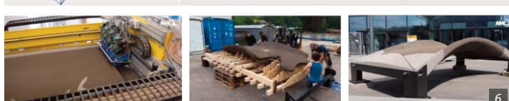
Figure 6. 3D printed pedestrian bridge: form finding, thickness optimization, segmentation, fabrication, installation and final result.
