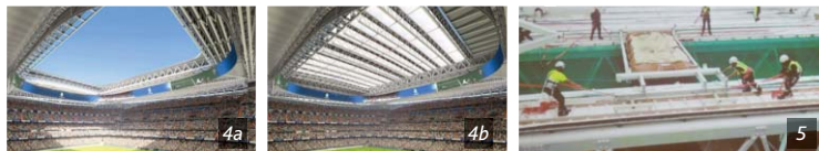
Figure 4a/b. The retractable roof open and closed.
