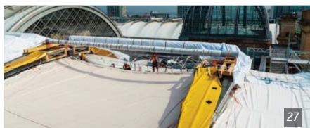
Figure 26. Palacio Nacional de Cultura, Guatemala, aerial view and detail. Figure 27. Renovation of Dresden Central Station membrane roof. Aerial view. Figure 28. Renovation of Dresden Central Station membrane roof. Installation.
