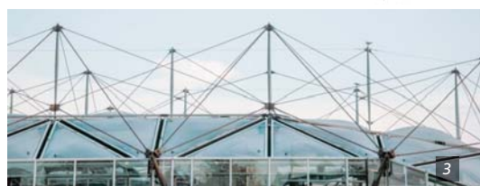
Figure 2. Drawings of the ETFE roof © Buitink Technology Figure 3. Detail of the facade and roof © ZJA Architects & Engineers
