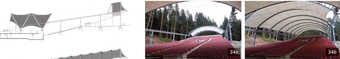
Figure 33. Retractable roof over the historic natural theatre in Bad Elster.
