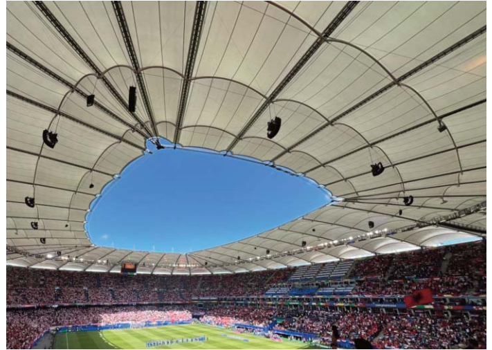
Figure 1. The renewed spoke-wheel membrane roof © sbp
