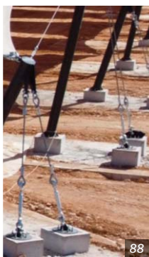
Figures 87-88. Antalya wholesale fruit market. The approach of snl tensi focused on: • High-strength steel cables and membrane materials, ensuring resistance to Antalya's high temperatures and strong winds. • Light and robust design, maximizing coverage while minimizing structural loads. Figure 89. Misir Mall of Arabia. Figure 90. Atakoy International Youth Centre, Istanbul. Figure 91. FIFA Dünya Kupası.
