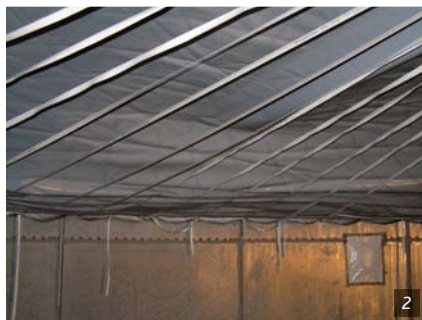
Figure 1. Example of a biogas storage system with membrane cover.
