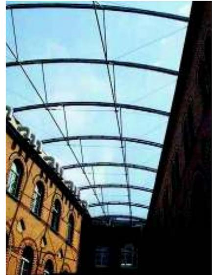
Figure 3. Ingenhoven & Partner, Architects, 2002: Kapuzinergräbe, Aachen. The Texlon® ETFE system accommodates a much larger range of structural movement than conventional cladding systems so that the overall structural weight is reduced by decreasing the stiffness.
