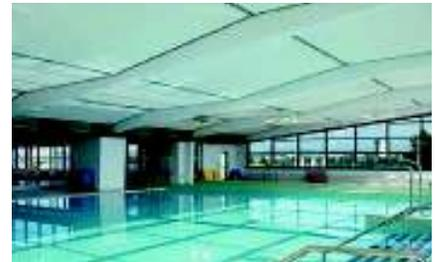
Figure 12. Batyline Aw and Silcord swimming-pool tensed ceiling.
