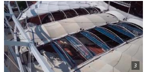
Figure 3: Replacement of the membrane roof of the Stuttgart Stadium.
