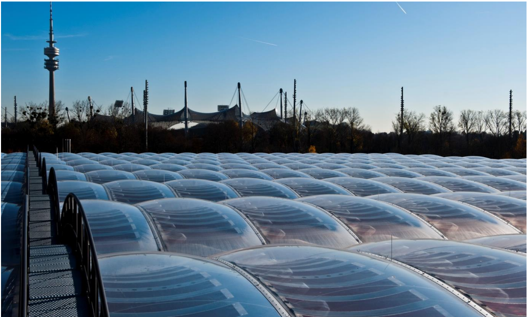
Figure 1:AWM carport-roof, top view
