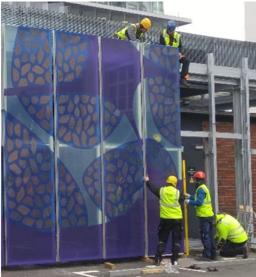
Figure 14: Installation of the pre-fabricated façade-modules on site
