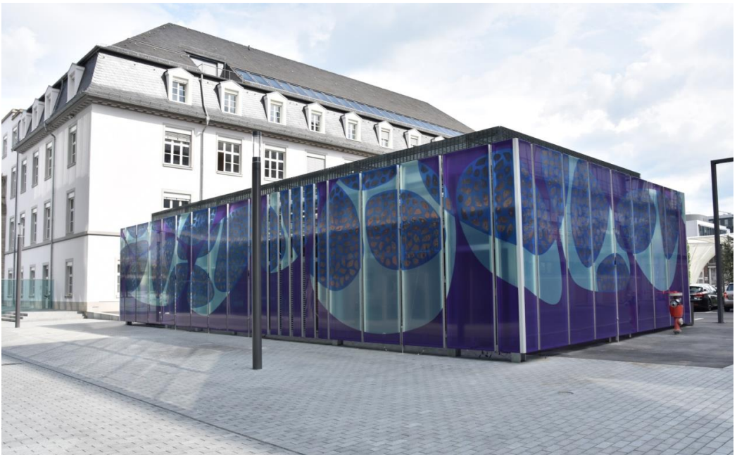
Figure 17:MERCK Transformer Station, Darmstadt, Germany: appearance of the new curtain wall
