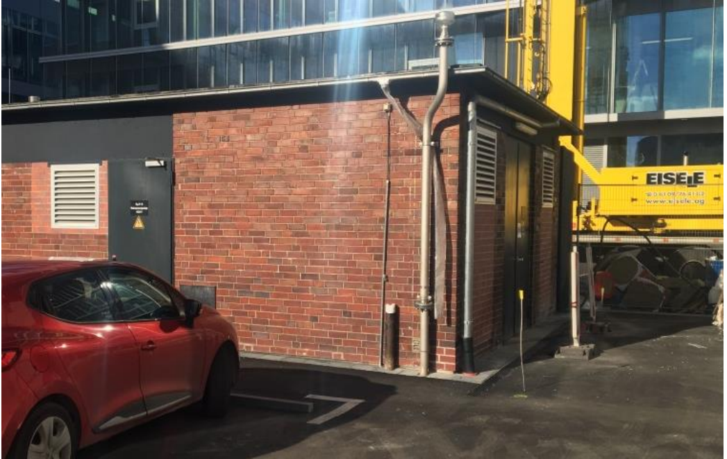
Figures 16:MERCK Transformer Station, Darmstadt, Germany: appearance of the original brick-façade
