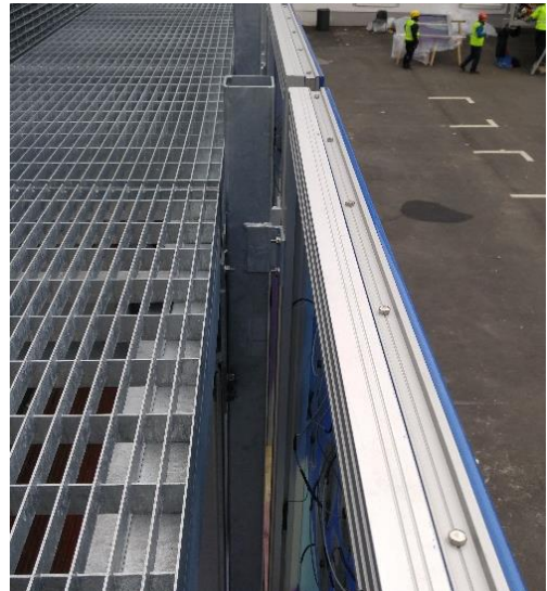
Figure 15: Finished façade (MERCK premises, Darmstadt, Germany)
