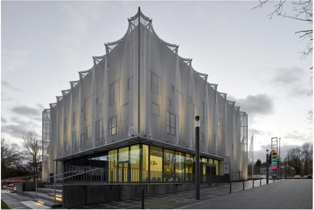
Figure 16: East and North façade
