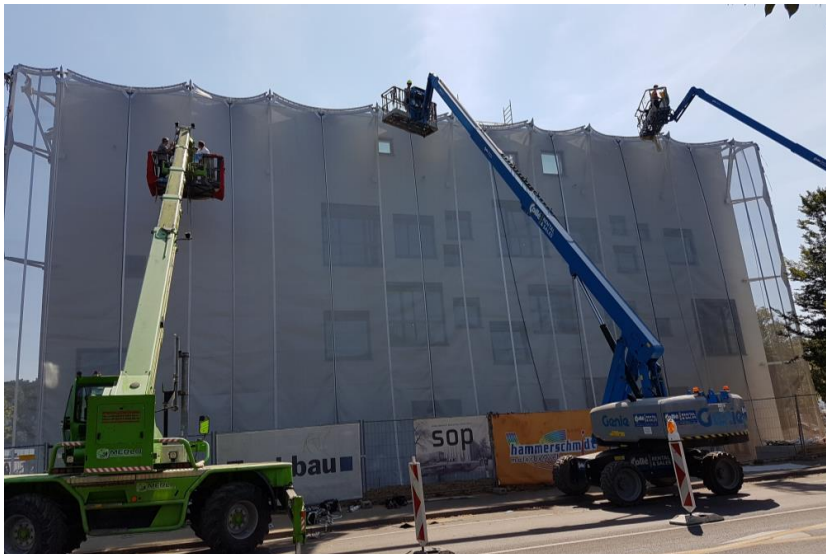
Figure 13: Attaching of the membrane panel
