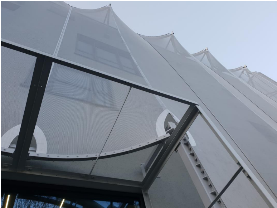
Figure 15: View from below at a door frame
