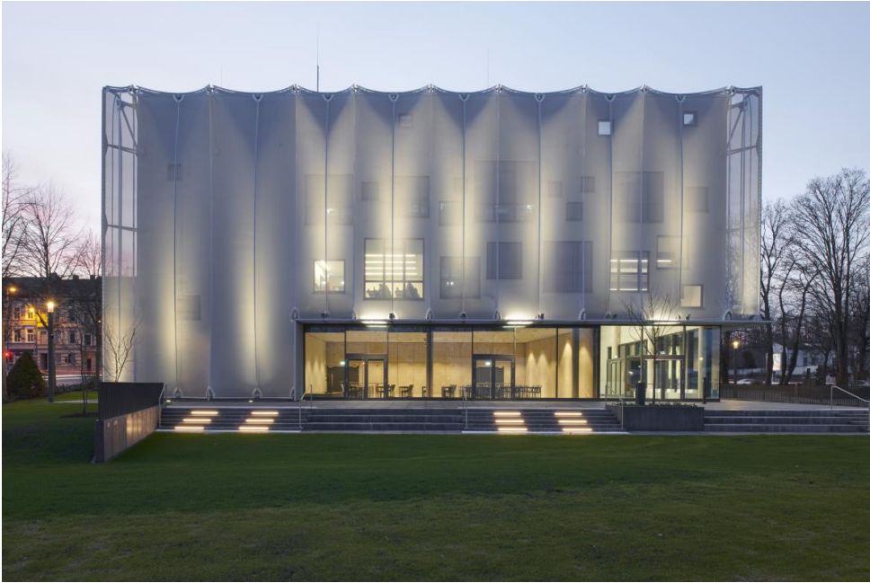
Figure 18: East façade in the twilight
