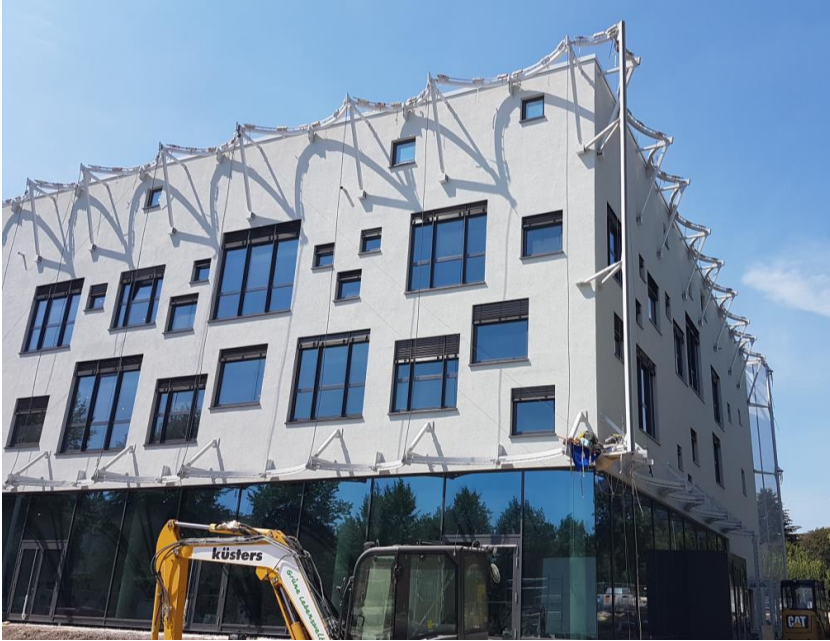
Figure 12: Support structure installed
