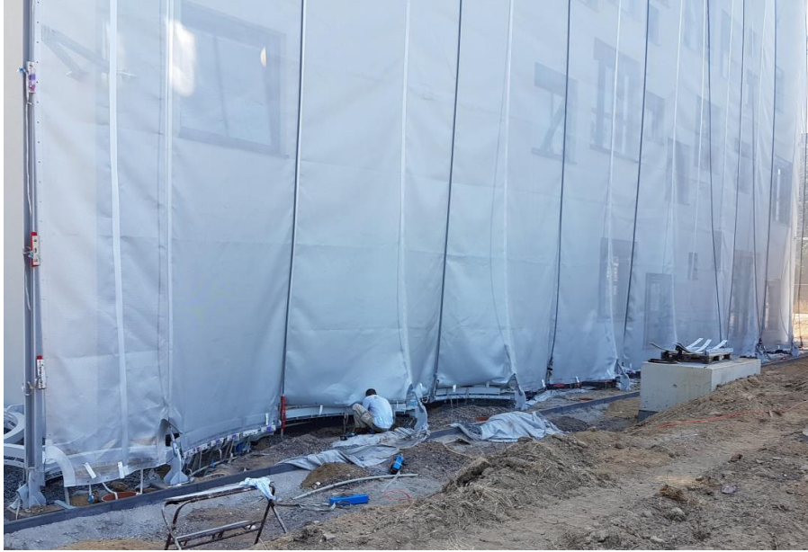
Figure 14: Stressing and fixing along the lower edge
