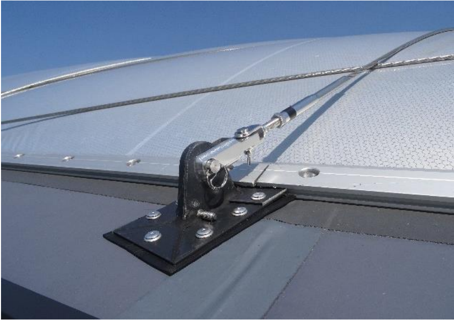
Figure 13: cable connection detail with printed upper cushion layer (formTL)
