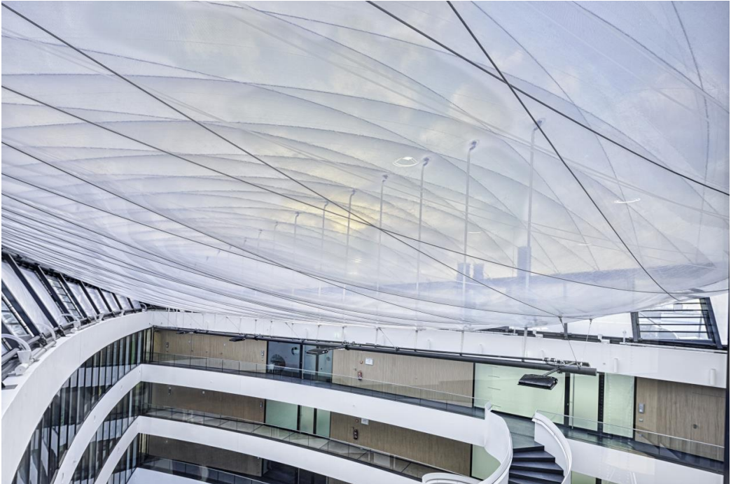
Figure 5: ETFE-cushion with stainless steel cable reinforcement (Hanno Keppel)
