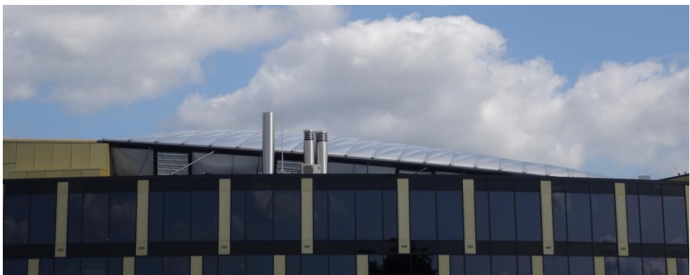
Figure 2: façade with ETFE-cushion-roof (formTL)
