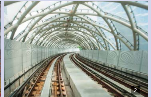
Figure 1a - b. The air tunnel encloses a curved section of the track with 363 film cushions, which are made from the high-performance 3M Dyneon Fluoroplastic ETFE © Architen Landrell Figure 2. The ETFE films for the roughly 2.500m 2 of exterior surface feature a smooth surface so that a rain shower is sufficient to clean them. That reduces the operational costs.
