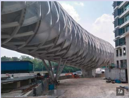
Figure 1a - b. The air tunnel encloses a curved section of the track with 363 film cushions, which are made from the high-performance 3M Dyneon Fluoroplastic ETFE © Architen Landrell Figure 2. The ETFE films for the roughly 2.500m 2 of exterior surface feature a smooth surface so that a rain shower is sufficient to clean them. That reduces the operational costs.
