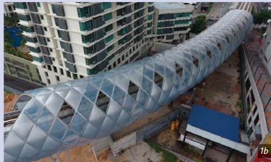
Figure 1a - b. The air tunnel encloses a curved section of the track with 363 film cushions, which are made from the high-performance 3M Dyneon Fluoroplastic ETFE © Architen Landrell Figure 2. The ETFE films for the roughly 2.500m 2 of exterior surface feature a smooth surface so that a rain shower is sufficient to clean them. That reduces the operational costs.
