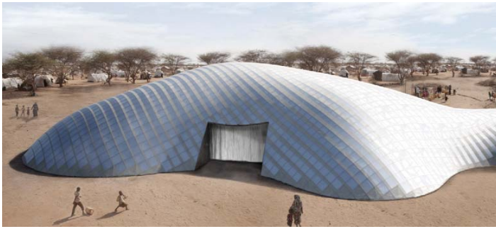
Figure 22. Rendering of a pneumatically erected elastic gridshell for a highly suitable application of the novel method: large-span, rapidly deployable disaster-relief or event shelter.
