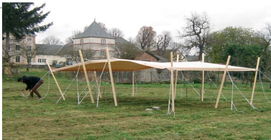
Figure 7. Prototype 2 - in search to optimise tensioning
