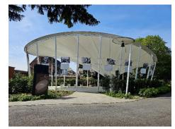
Located in the southern cemetery of Tournai, the multi-philosophical space is designed to host respectful farewell ceremonies. This semi-open space is covered by a white tensioned membrane. The space is oval, the stretched membrane is fixed on a ring supported by twenty posts and lowered in one place. The floor, made of a very light, smooth concrete, is also elliptical. It covers 215m<sup>2</sup>. The project has a contemporary and refined touch and respects its environment.
