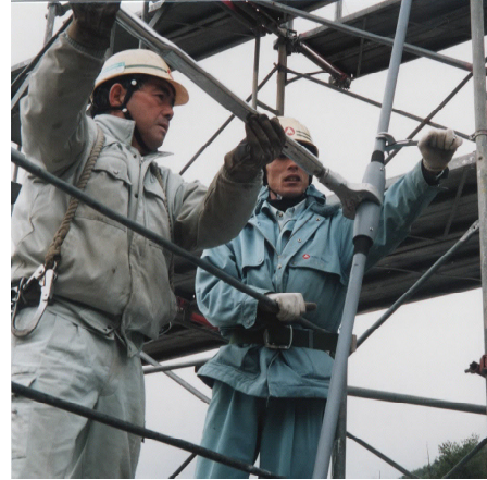
(b) Manual prestressing process
