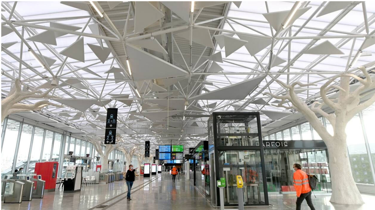
Figure 4. The new 'mezzanine' with a polycarbonate roof, ©Jérôme Fouquet/Ouest-France
