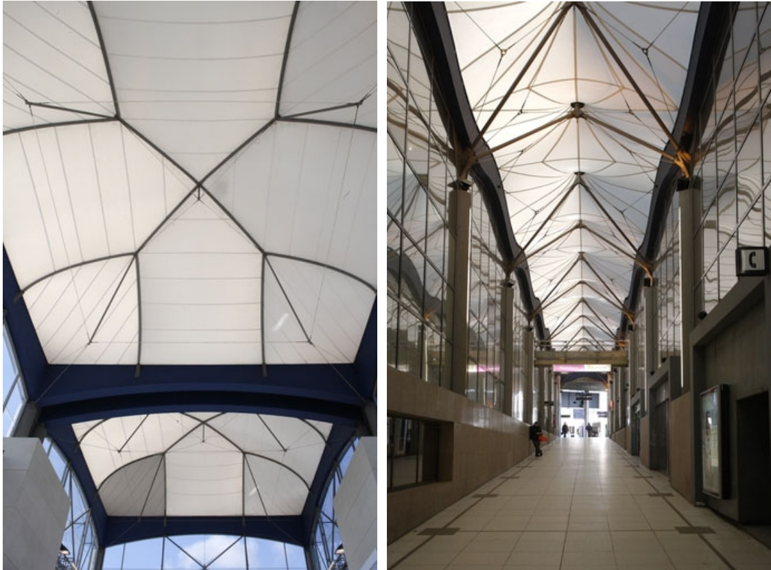
Figure 2. Textile roof from the inside, ©Pillet Denis
