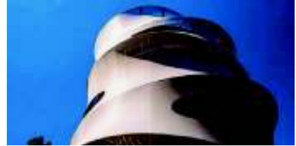
Figure 21. Textile façade of the Velaa Island restaurant
