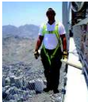
Figure 17. X-TEN mesh as exterior scaffolding
