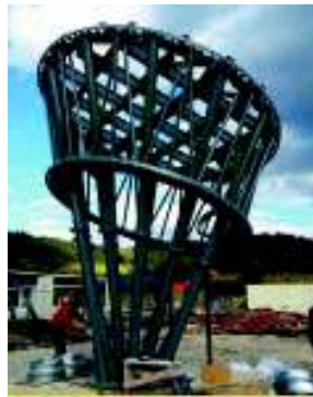
Figure 20. The high "point" of the Gino Park membrane before erection
