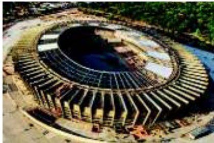
Figure 10. gmp Architekten, 2014: Mineirao Stadium under construction, Belo Horizonte
