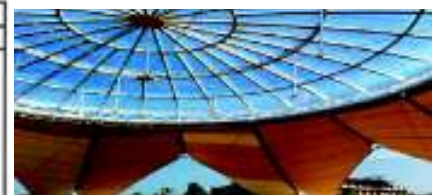
Figure 14. ETFE in China: Sun Island membrane structure, Heilongjiang (Seele Covertex Membranes Shanghai Co.)
