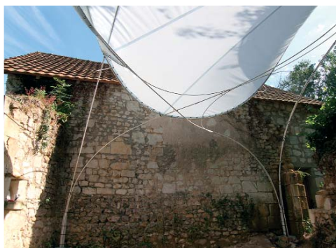
Fig 8a-c: Individual components of the hybrid system: Bending-active GFRP Structure, attached form-active textile membrane, internal cell structure.
