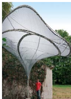
Fig 9a-d: The textile hybrid M1: Internal view of multilayer membrane system with integrated cells. External view in the context of the tower ruin.
