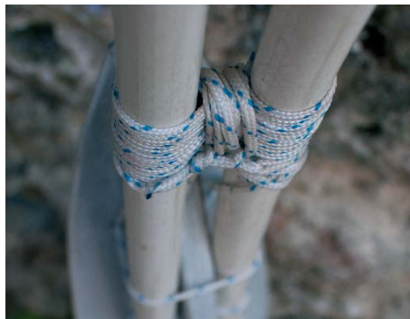
Figure 7a-b: Lashing details for the GFRP rod assembly
