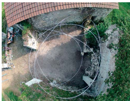
Fig 8a-c: Individual components of the hybrid system: Bending-active GFRP Structure, attached form-active textile membrane, internal cell structure.
