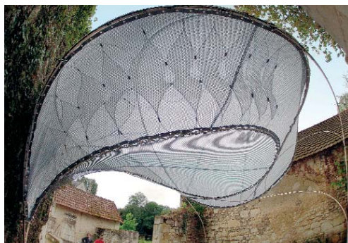
Fig 9a-d: The textile hybrid M1: Internal view of multilayer membrane system with integrated cells. External view in the context of the tower ruin.
