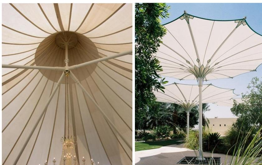
Figure 6-1 Membranes partly reinforced with a second layer: at the high point (left) and at the low point and membrane corners (right)
