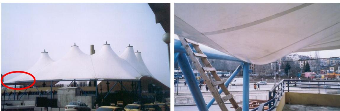
Figure 7-1 Ponding at the corner of conic structures caused by rain load in combination with rotating of the pylons (kinematics displacement) of the supporting structure, Central Railway Station Square, Sofia [© V. Tanev]
