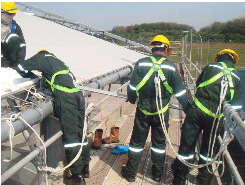
Figure 2. Attaching the membrane to the frame, from https://temembrane.com/portfolio-item/installation/
