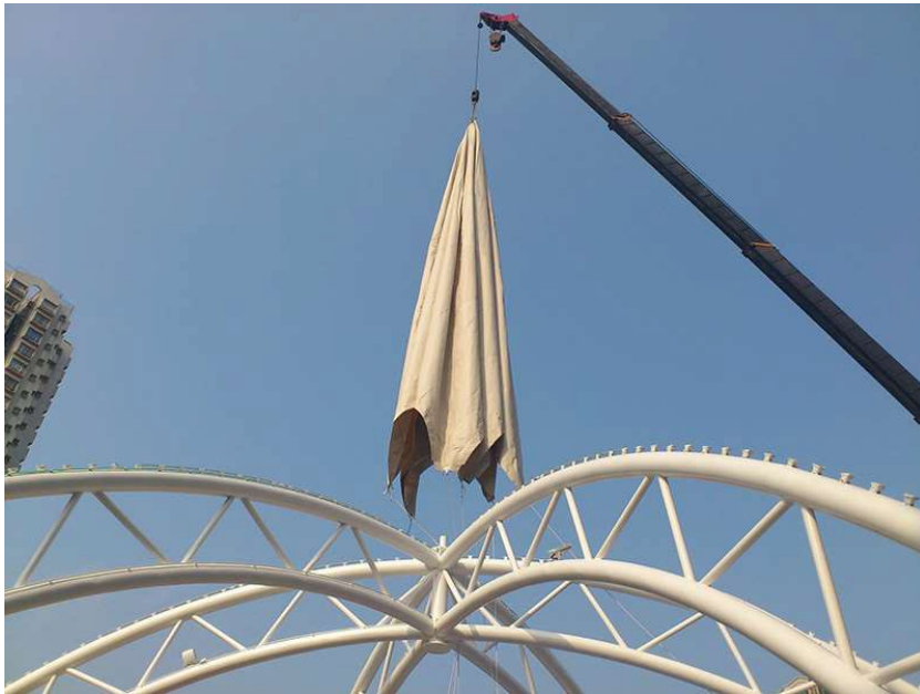
Figure 1. Installing the membrane, from https://www.cantensile.com/garden-park-architectural-ptfe-tensile-structure-pavilion_p31.html
